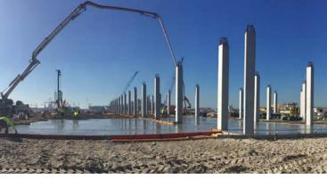
**CONSTRUCTION** work on Brisbane's new International Cruise Terminal is proceeding apace, with almost all of its 107 wharf piles installed and major civil works including concrete pours and the base of the new terminal building in progress.
